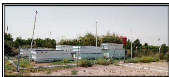
Fig. 2: Constructed wetland systems station at Basrah University
